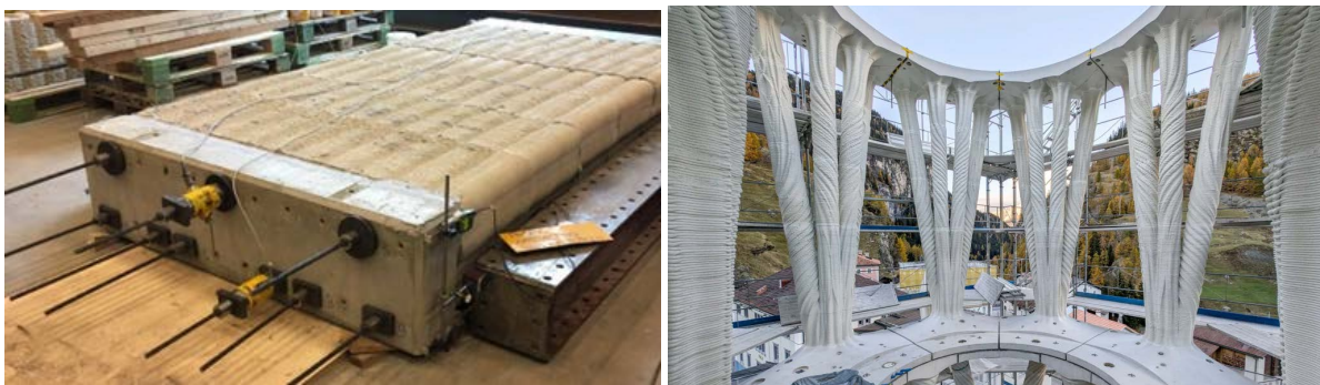
Figure 4.4: On the left the post tensioned bridge elements of the 3D-printed bicycle bridge in the Netherlands. On the right, the columns of the upper levels of the Tor Alva tower are post-tensioned using a central high-tension steel bar ( \varnothing 12 mm). These bars are greased and housed in plastic sleeves, with their anchorages integrated into the prefabricated concrete elements [86].
