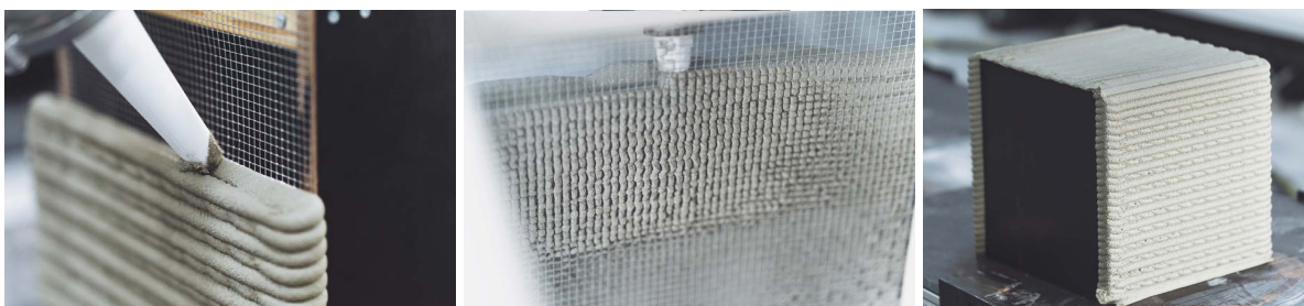
Figure 4.7: 3D concrete printing directly onto pre-assembled wire-frame reinforcement structures by Vertico [89].
