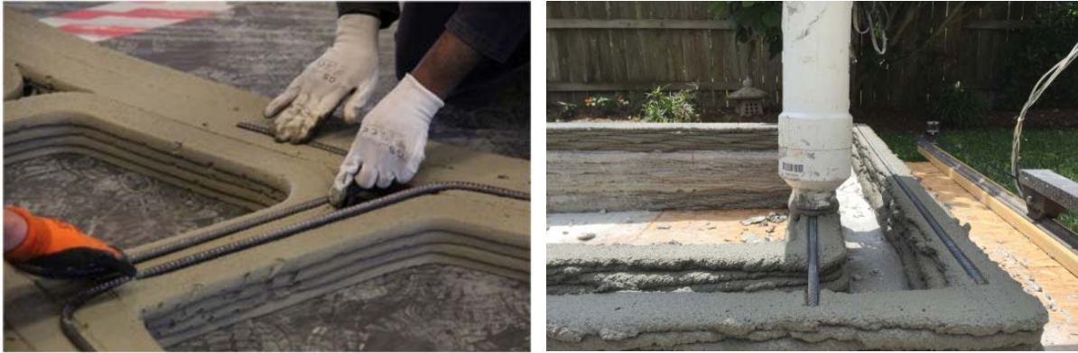
Figure 4.14: Examples of reinforcement strategies in extrusion-based 3D concrete printing. (left) Demonstration of placing reinforcement between layers during fabrication at TU Eindhoven, enabling contiguous in-layer strengthening along the printing path; (right) Integration concept illustrated by the V2 Vesta concrete 3D printer, adapted from [99].
