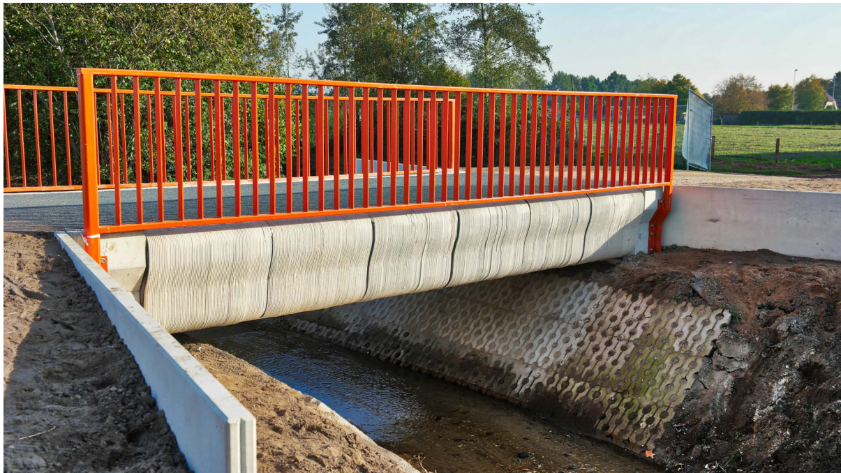
Figure 3.17: 3D concrete printed bridge in Gemert
