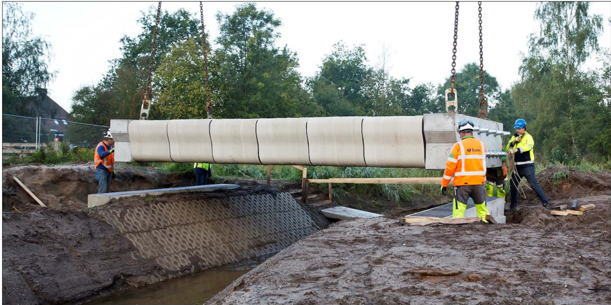
Figure 3.18: Gemert bridge assembly
