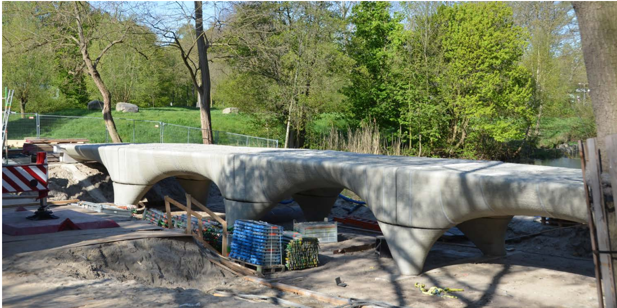
Figure 3.25: Multiple girders assembled, courtesy De Gelderlander (Paul Rapp)
