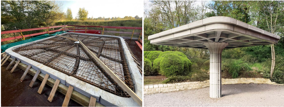
Figure 4.10: Printed formwork demonstrator developed at Technische Universität Darmstadt.
