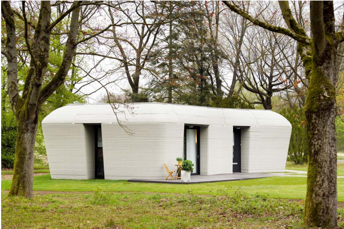
Figure 3.26: The first house of project Milestone
