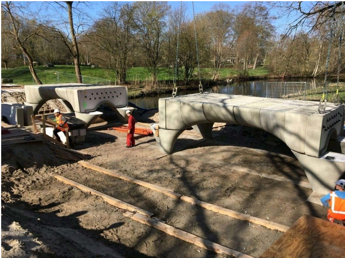
Figure 3.20: The five prestressed girders being assembled on site in Nijmegen
