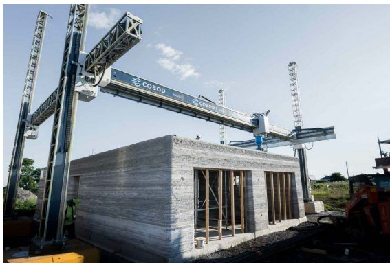
Figure 3.2: Examples of Cartesian gantry-type 3D concrete printers. Left: a COBOD system configured for full-scale on-site printing [51]. Right: large-scale gantry at TU/e 3DCP research laboratory
