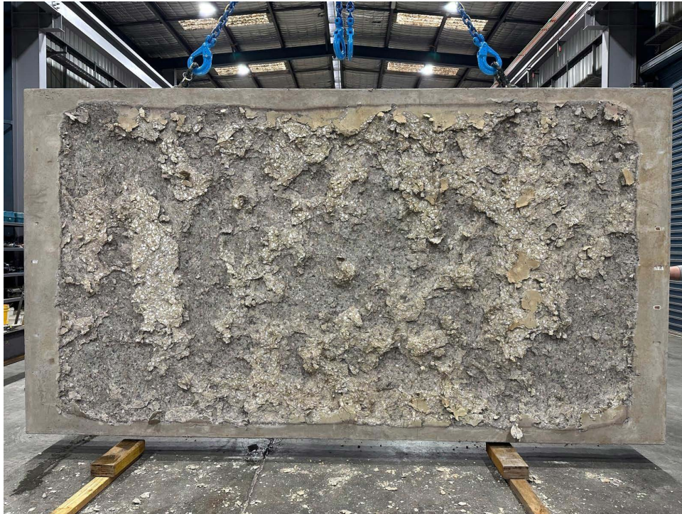
Figure 2.8: Spalling in a 4400×2400×400 mm reinforced concrete wall subjected to a high compressive stress was exposed to a modified hydrocarbon fire, measured local losses exceeding 100 mm in depth.
