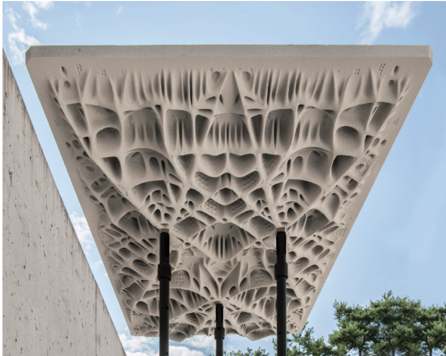
Figure 2.10: Topology optimization of a slab with three supports, taken from [10].
