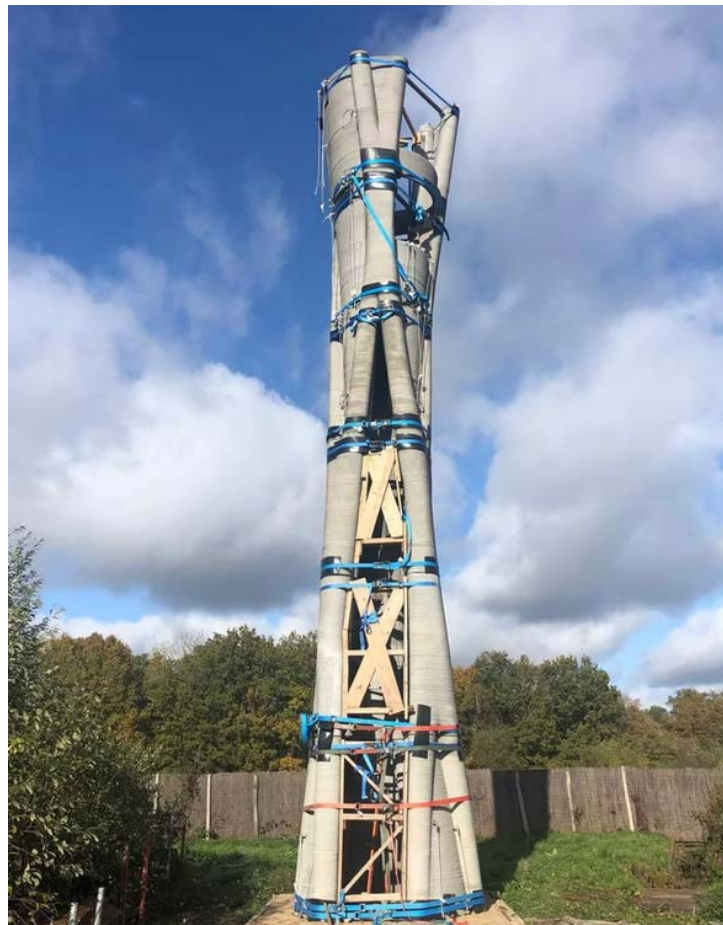
Figure 5.19: XtreeE telecommunication mast. Taken from [56].
