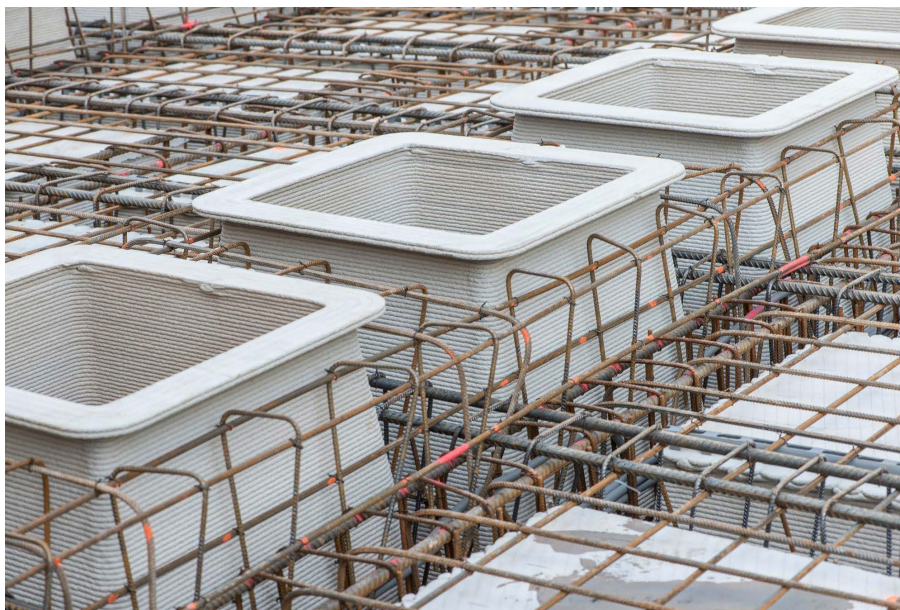
Figure 5.8: Sky lights are placed in the slab. [51].
