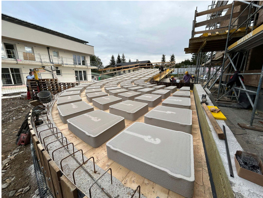
Figure 5.2: Bauminator bended slab. Taken from [47].
