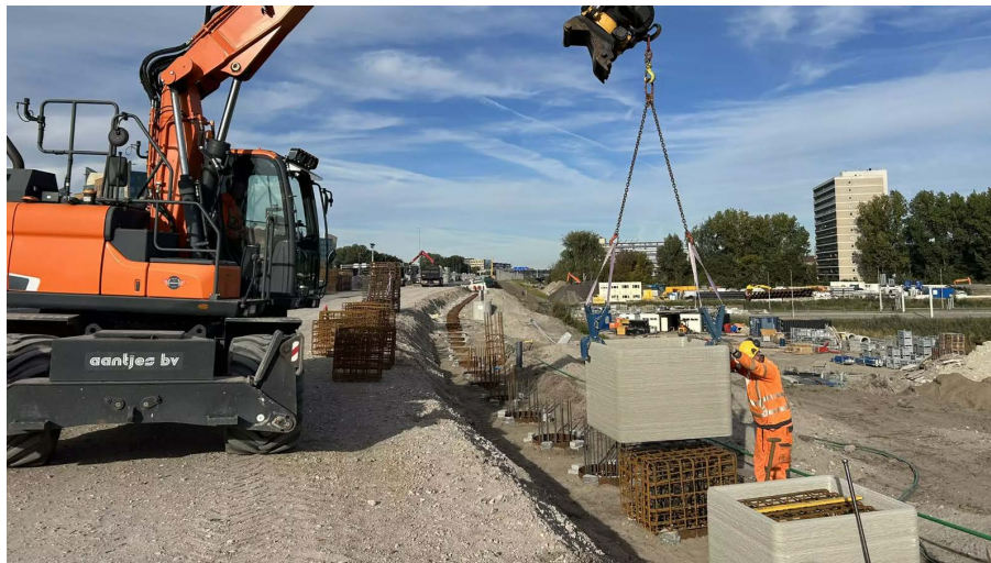
Figure 5.14: Placement of 3D concrete printed foundation block lost/stay-in-place formwork. Taken from [54].
