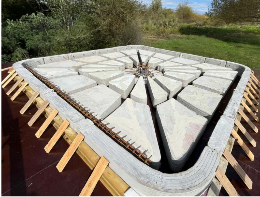
Figure 5.17: Assembly on-site. Taken from [55].
