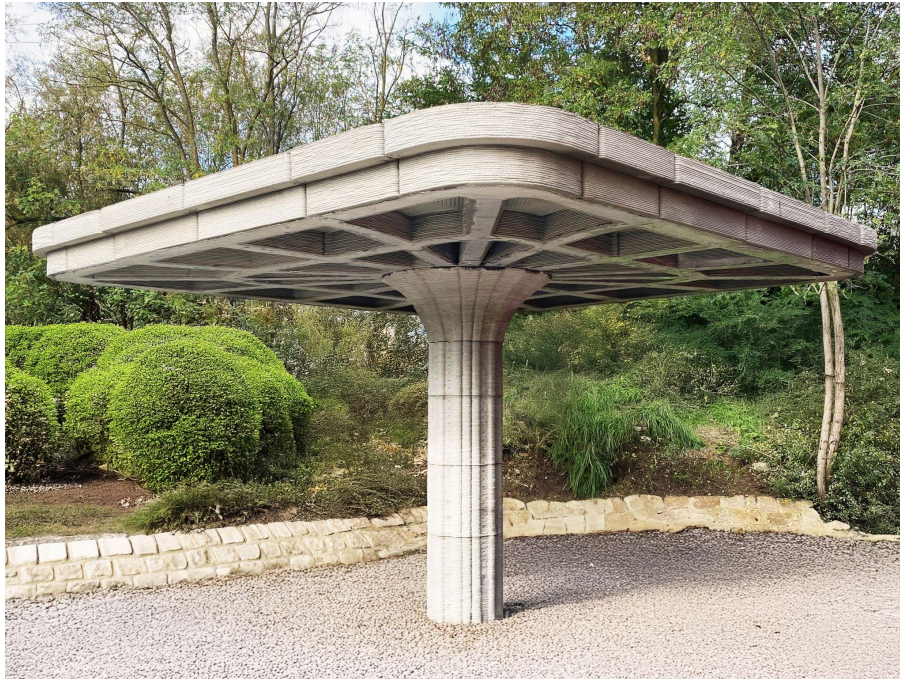
Figure 5.16: Mushroom column-supported canopy, made by Riedel Bau Firmen-gruppe, in collaboration with TU Darmstadt. Taken from [55].
