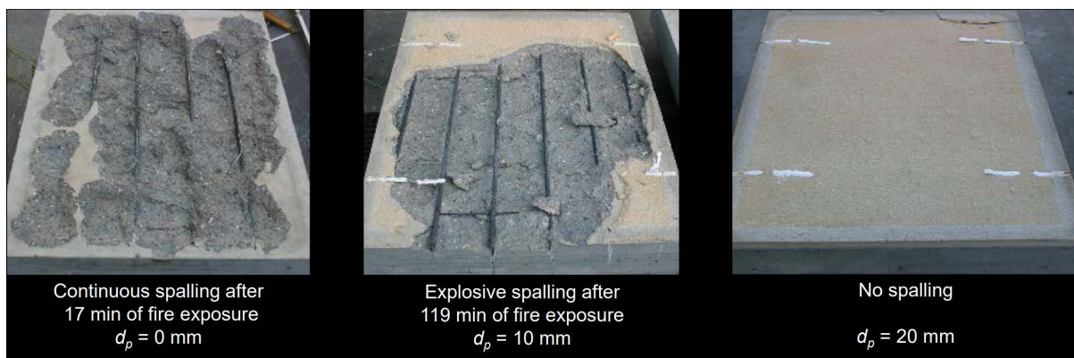
Figure 2.7: Image taken from the Advanced Structural Concrete lecture series of ETH Zurich [5], based on experimental fire tests originally reported by Klingsch [6].
