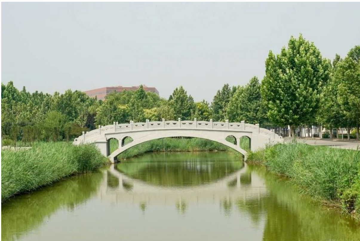
Figure 5.9: 3D Concrete printed bridge at the campus of Hebei University of Technology, China. The bridge design is inspired by the Anji Bridge, located in Zhaoxian county (built around 581-618). Taken from [53].
