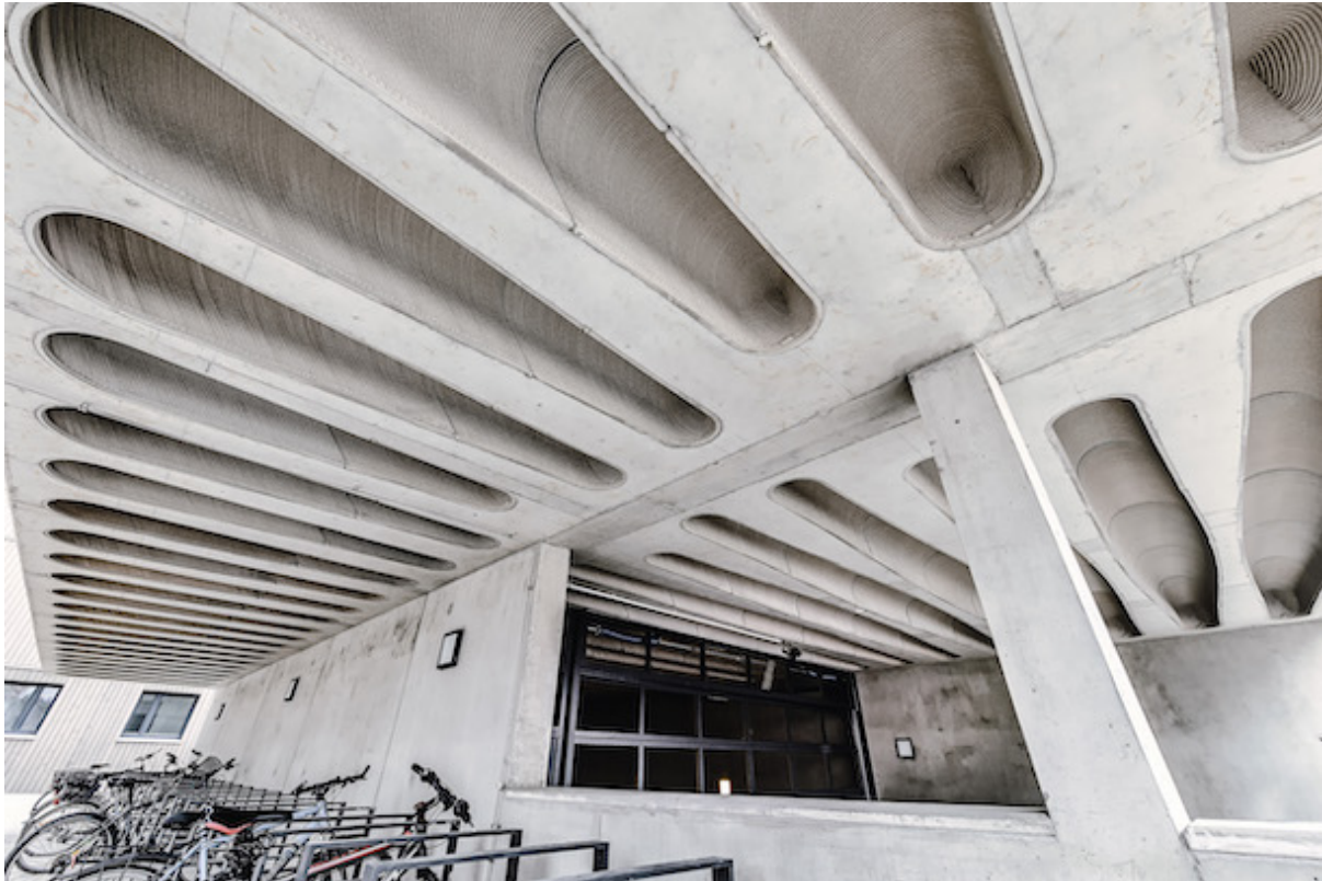
Figure 5.3: Parking Garage Entrance Nördlingen. Taken from [48].
