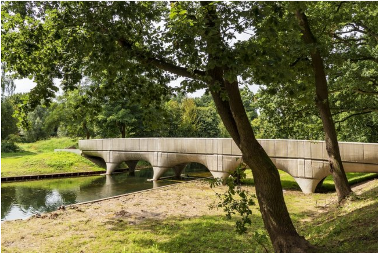
Figure 5.21: 3D concrete printed bicycle bridge in Nijmegen. Taken from [57].
