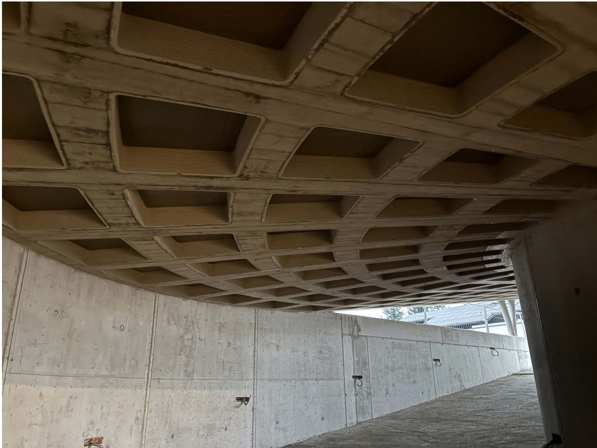
Figure 5.1: Parking garage entrance.
