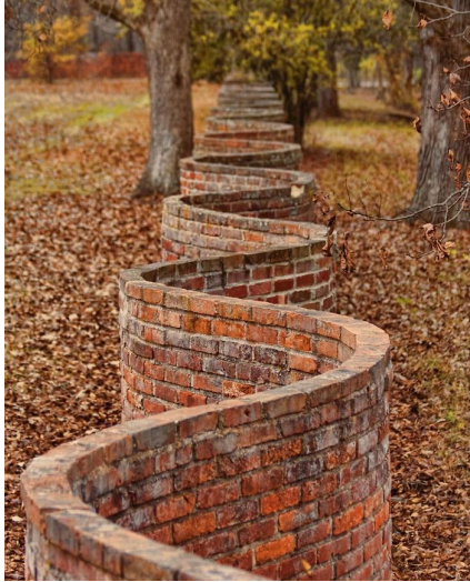
Figure 3.2: Comparison of traditional crinkle-crankle wall (left) and a digitally fabricated wavy 3DCP wall (right). Crinkle-crankle wall: a traditional wavy brick wall design that achieves stability through its serpentine form while using fewer bricks compared to a straight wall. Courtesy to [34]. Wavy 3DCP wall: parametric concrete wall form generated using computational design. Courtesy to [35].
