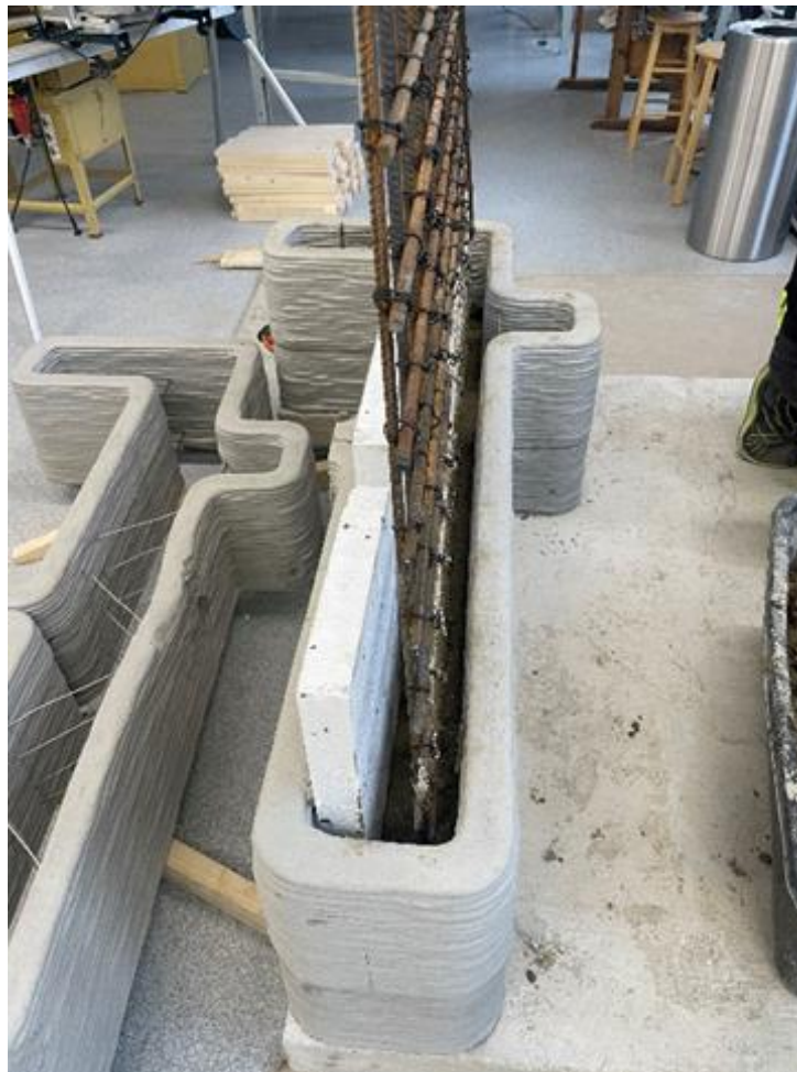
Printed wall element for experimental 3D printed cellar
